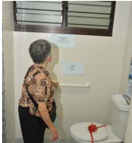
Improvements to the toilets.
