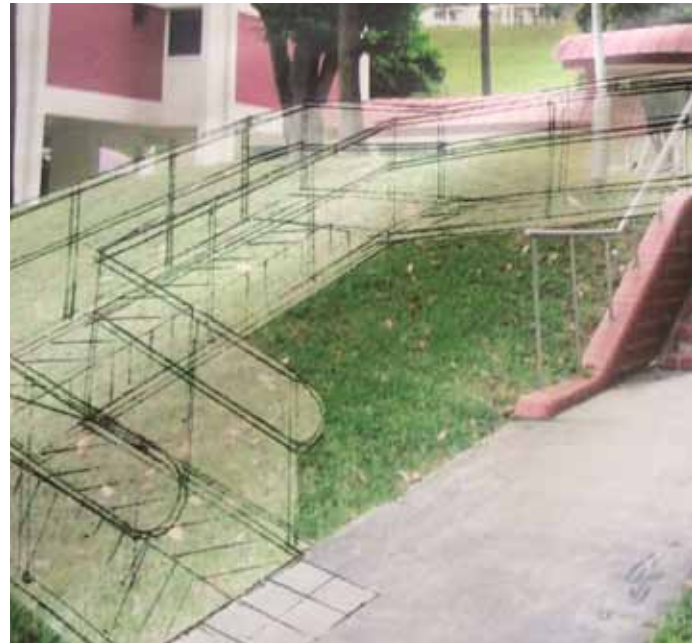
Blk 179 to carpark at Ang Mo Kio Ave 5
